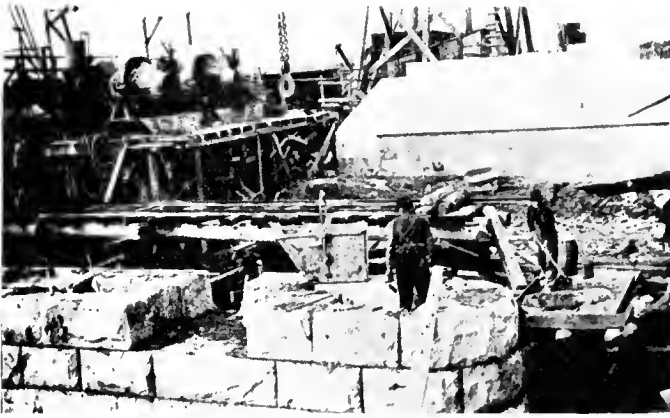
Fig. 2.— Pier B and north abutment.
